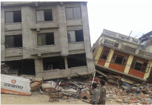
Fig. 1. The soft first stories collapsed in 2015 Gorkha Earthquake Nepal.
