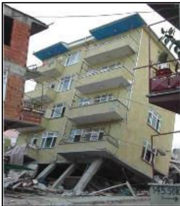
Fig. 1. Soft first story collapse in Golcuk, Turkey during the 1999 Turkey earthquake (source: Ahmet Topcu).
