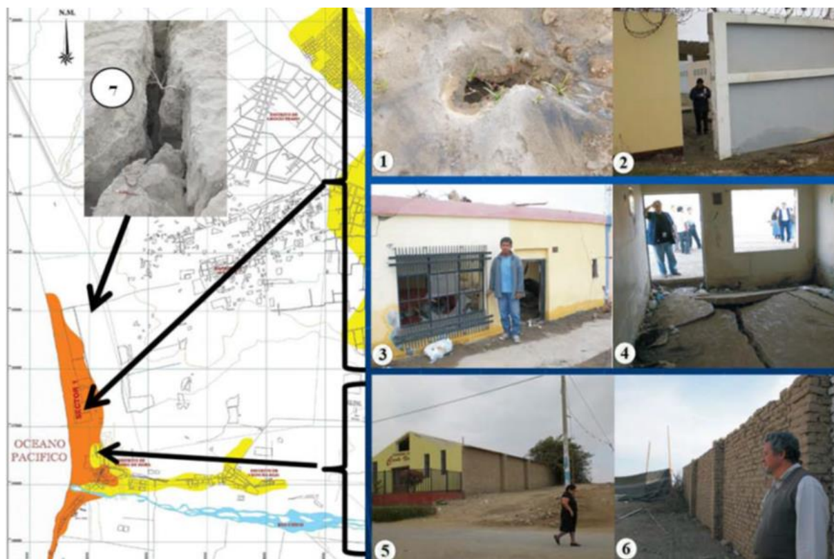
Fig. 7. Microzonation effects in Tambo de Mora and photos taken in August, 2007 after the Earthquake of August 15, 2007. (1) Volcano of soil liquefaction. (2) Lateral spreading, a “door was opened”. (3) Settlement of 0.80m 1.00m. (4) Settlement of bearing walls and broken concrete floor. (5) Undamaged adobe church. (6) Adobe fence, only 200 m from the Tambo de Mora main square (Plaza de Armas) where soil liquefaction occurred. (7) Large and abundant cracks were opened north of Tambo de Mora where also a 3 km long and 0.6 km wide block was displaced a few meters toward the ocean. Microzonation map is a courtesy of INDESI. All photos are taken by the author.
